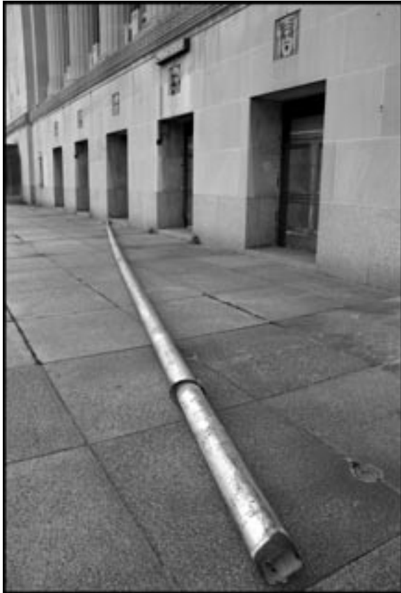
PIPE, ST. LOUIS, MO. PHOTOGRAPH BY ROGER PFINGSTON.
